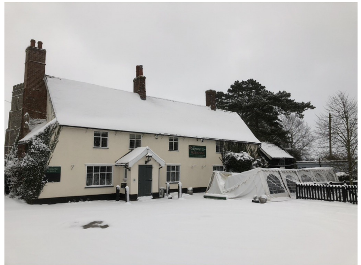
The collapsed marquee at “The Greyhound” on 8 th February.
